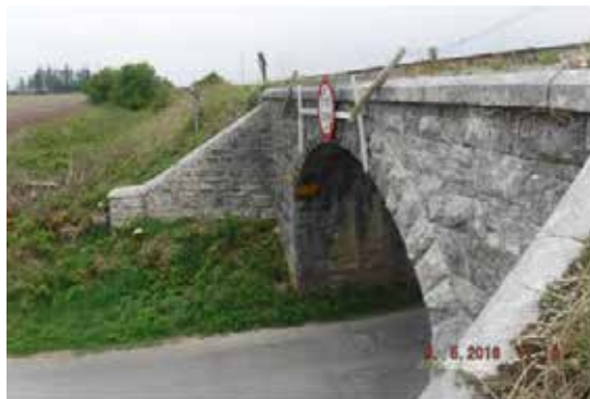
Figures 5.14 and 5.15 are close-up views following vegetation clearance of the wing walls of UBE180 (at milepost 65 miles 1220 yards). Down-side (l) and up-side (r). This structure is in good condition. (Courtesy of Iarnród Éireann).
