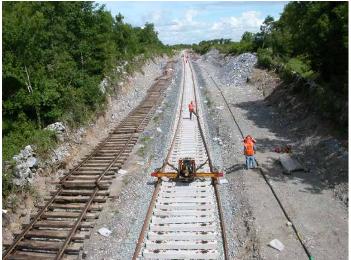
Figure 3.2: Phase 1: New track being laid during renewal of Ennis-Athenry (P. Newman)
