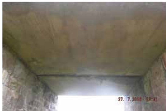
Figures 5.22 and 5.23 are views of cattle pass UBE212 (at milepost 4 miles 1520 yards). Concrete deck with masonry abutments. (Courtesy of Iarnród Éireann).
