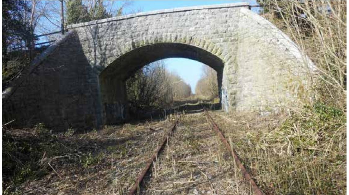
Figure 5.10 is a view looking towards Tuam of bridge OBE176 (at milepost (at milepost 63 miles 1617 yards) following vegetation clearance. It carries the public road R339 across the railway in Caraun, county Galway. This well-built bridge is a protected structure (NIAH No. 30407114 and RPS 3745) and was built in 1860. It is in good condition. (Courtesy of Iarnród Éireann).
