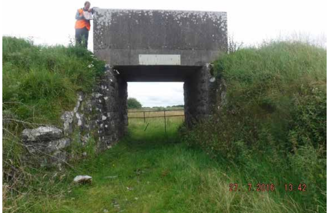
Figure 5.21 is a view of cattle pass UBE212 (at milepost 4 miles 1520 yards). (Courtesy of Iarnród Éireann).
