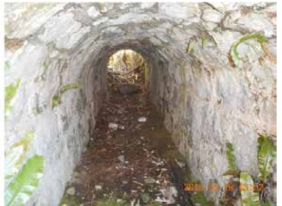
Figures 5.5 and 5.6 are views from down side showing the entrance and internal view of culvert UBE173A (sheep pass). The shape is good and condition is fair. (Courtesy of Iarnród Éireann).
