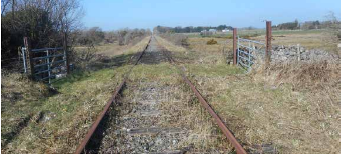
Figure 5.7 is a view across level crossing XE212 (f-type) (at milepost 63 miles 0876 yards) looking towards Tuam. (Courtesy of Iarnród Éireann).
