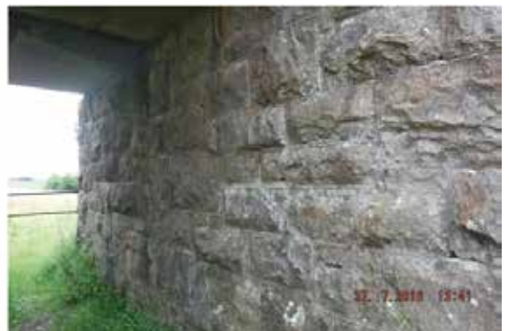
Figures 5.22 and 5.23 are views of cattle pass UBE212 (at milepost 4 miles 1520 yards). Concrete deck with masonry abutments. (Courtesy of Iarnród Éireann).
