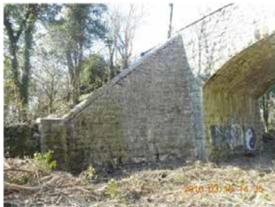
Figures 5.11 and 5.12 are close-up views following vegetation clearance of the wing walls of OBE176 (at milepost 63 miles 1617 yards). Down-side (l) and up-side (r). This structure is in good condition. (Courtesy of Iarnród Éireann).
