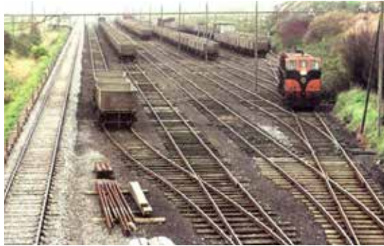
Figure 2.10: Former Sugar Factory sidings Tuam 1975 (Pic. David Carse)
