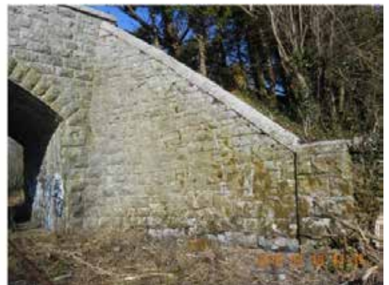
Figures 5.11 and 5.12 are close-up views following vegetation clearance of the wing walls of OBE176 (at milepost 63 miles 1617 yards). Down-side (l) and up-side (r). This structure is in good condition. (Courtesy of Iarnród Éireann).
