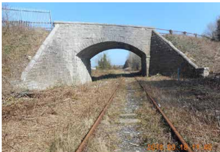
Figure 5.2 is a view looking towards Tuam of bridge (OBE168) (at milepost 60 miles 1724 yards) following vegetation clearance and minor re-pointing works in 2016. It carries a public road in Caherroy, Athenry. This well-built bridge is a protected structure (NIAH No. 30332005 and RPS 3972) and was built in 1860. It is in good condition. (Courtesy of Iarnród Éireann).
