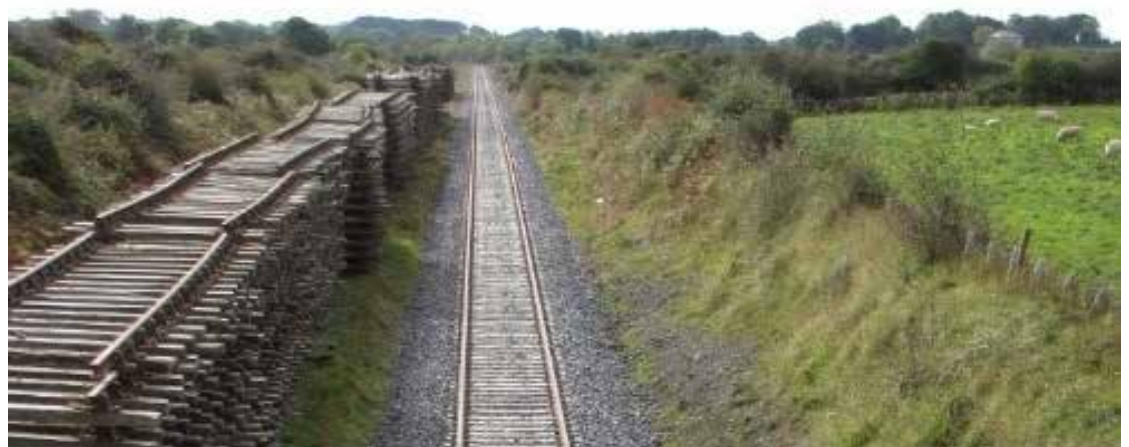
Figure 5.29 Old track awaiting disposal alongside the new alignment between Ennis and Athenry (P. Newman).
