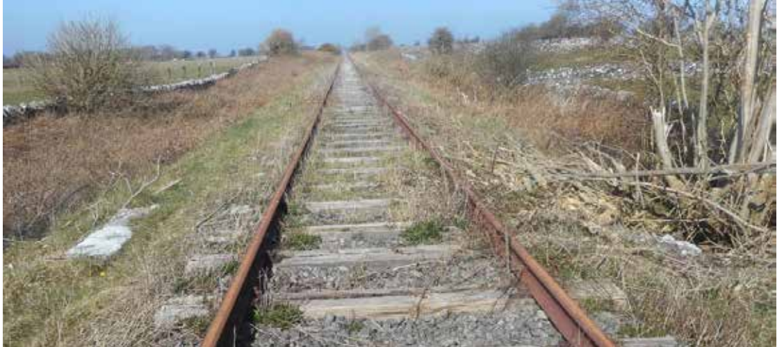
Figure 5.4 is a view across culvert UBE173A (at milepost 62 miles 0528 yards) looking towards Tuam. (Courtesy of Iarnród Éireann).
