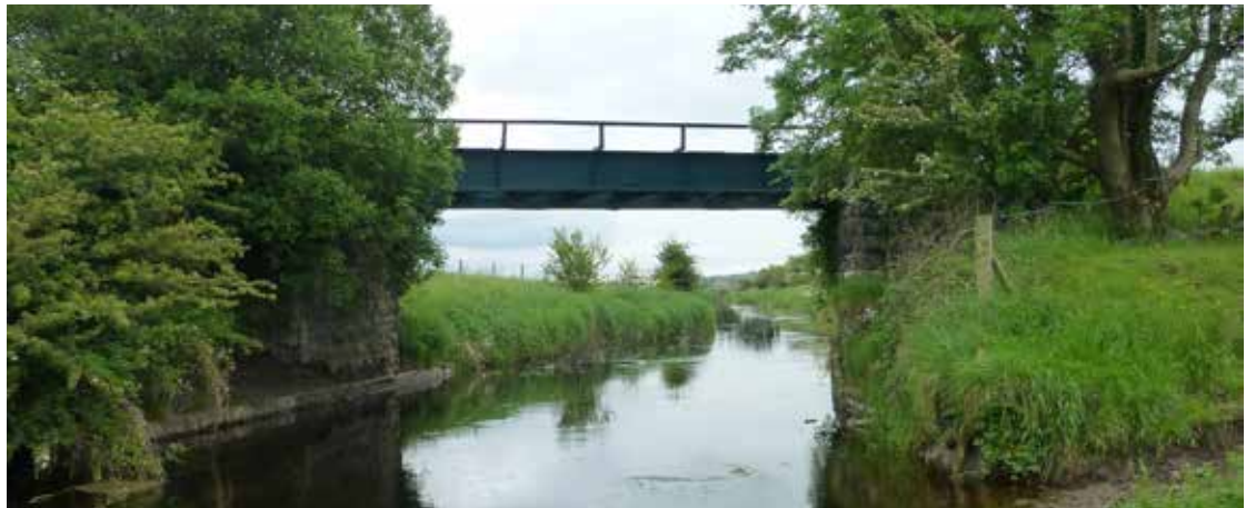
Fig 5.16b Looking east (upstream) at Abbert River bridge just south of Ballyglunin, at MP 69 miles 1300 yards. The steelwork on this bridge is in good condition as it was painted in 2002 to protect it from deterioration. (P. Bowen Walsh)
