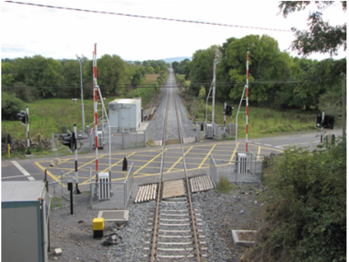
Fig 5.30 A new CCTV level crossing at N18 Kiltartan on Phase 1 (A Mogridge).
