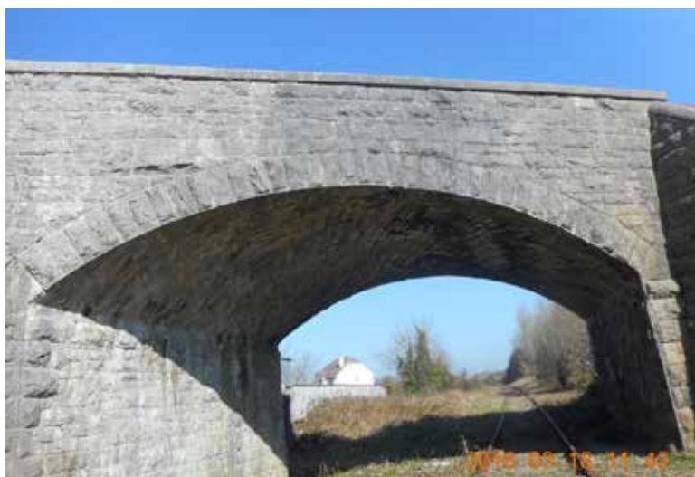
Figure 5.3 is a closer view of OBE168 (at milepost 60 miles 1724 yards) following vegetation clearance and minor re-pointing works. This skew-arch soffit shows some water staining but is in good condition. (Courtesy of Iarnród Éireann).
