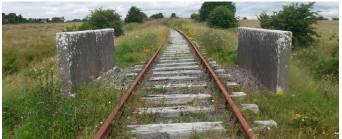
Figure 5.20 is a view towards Claremorris across cattle pass UBE212 (at milepost 4 miles 1520 yards). Fair condition. (Courtesy of Iarnród Éireann).
