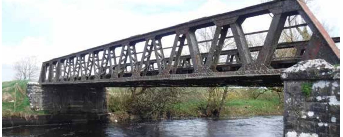
Figure 5.16a (at milepost 1 mile 1520 yards) is a major steel truss-type bridge (UBE206) of 20m span across the River Clare near Tuam. This structure has potential to be renovated and re-used. (Courtesy of Iarnród Éireann).
