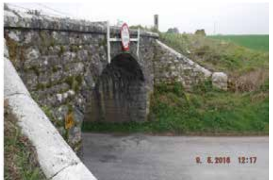
Figures 5.14 and 5.15 are close-up views following vegetation clearance of the wing walls of UBE180 (at milepost 65 miles 1220 yards). Down-side (l) and up-side (r). This structure is in good condition. (Courtesy of Iarnród Éireann).
