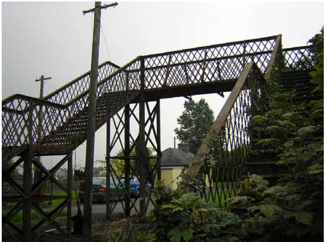
Fig 5.25 is bridge OBE222 at 16 miles 1270 yards, a pedestrian footbridge at Lower James Street, Claremorris. (E O'Boyle)
