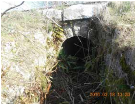
Figures 5.5 and 5.6 are views from down side showing the entrance and internal view of culvert UBE173A (sheep pass). The shape is good and condition is fair. (Courtesy of Iarnród Éireann).
