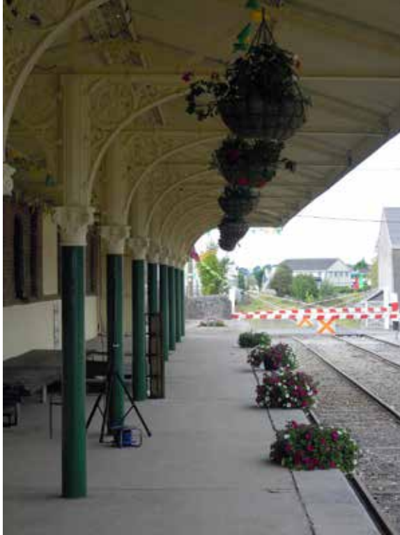
Figure A3.1 Tuam Railway Station (J. Canney)
