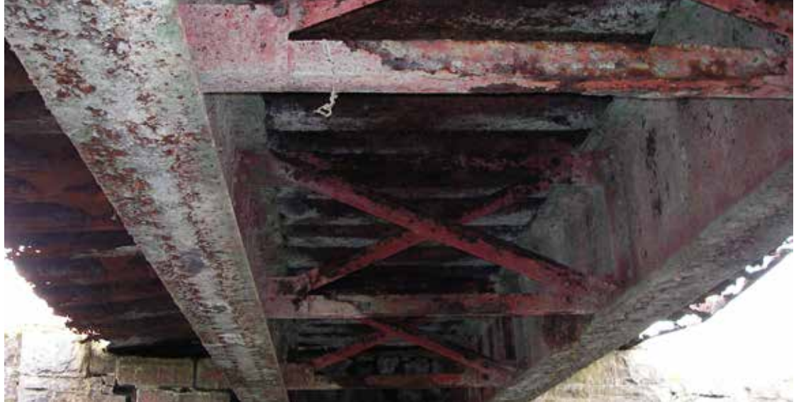
Figure 6.18 Underside of deck of trough girder steel Mullaghanoë River bridge (248) between mileposts 23.75 & 24.00
