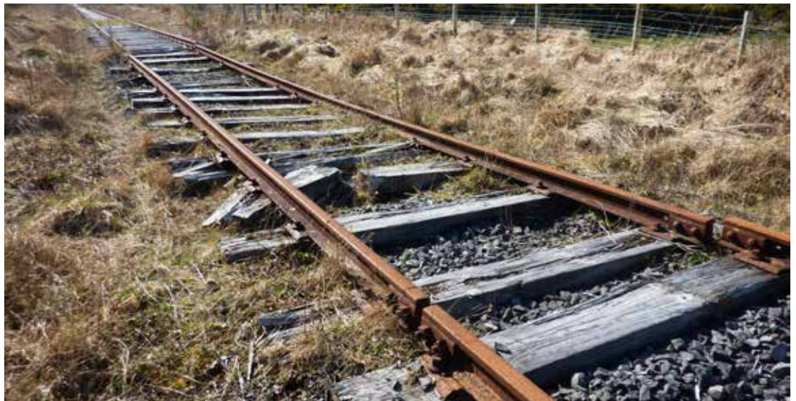
Figure 6.16 Apparent attempt to remove 30-foot length of track between Drumshinnagh level crossing and milepost 20.25
