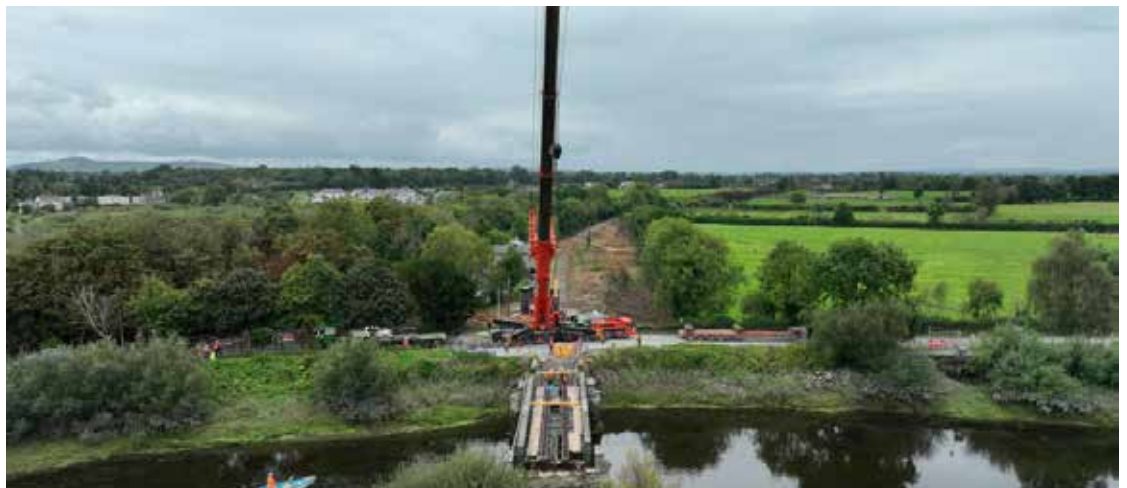
Figure 5.10: River Maigue Bridge at Adare being lifted out for renovation and restoration as part of the Limerick to Foynes Rail Project
