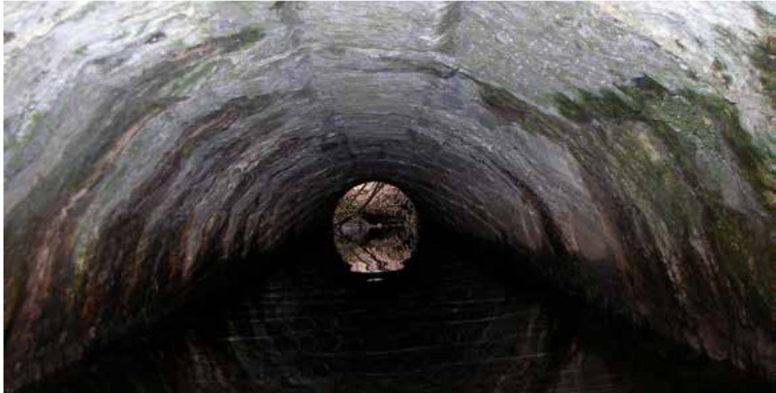
Figure 6.34: Unnumbered stone culvert in excellent condition, northeast of milepost 41.25.
