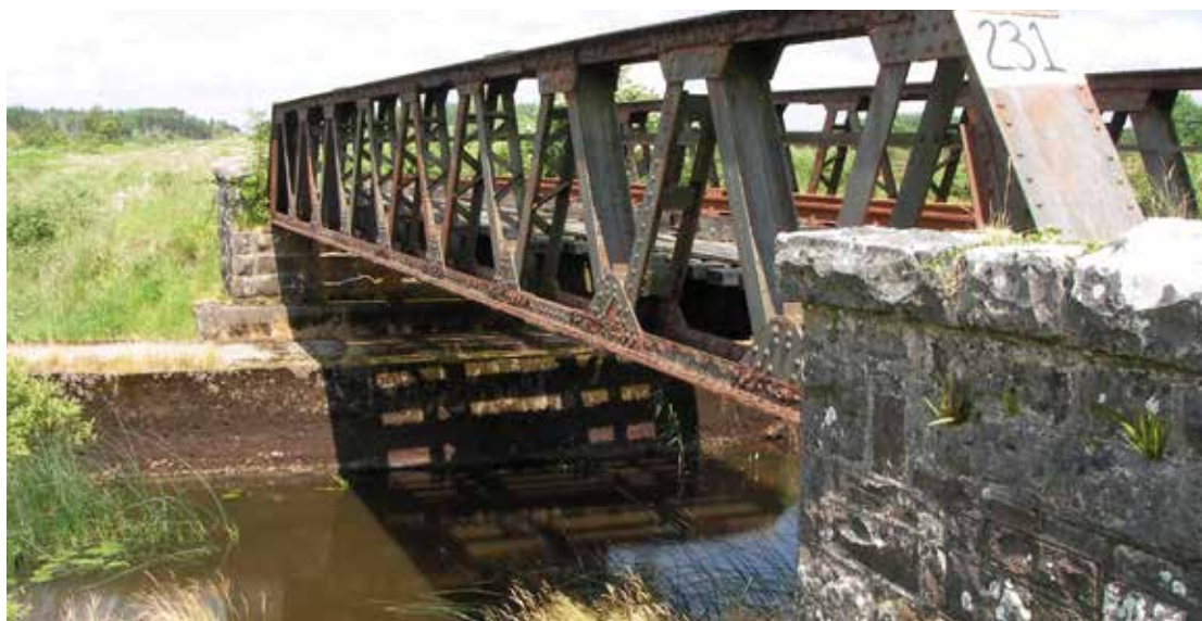
Figure 6.8: Single span Warren truss steel Girder Bridge UBCL 231 crossing the Yellow River
