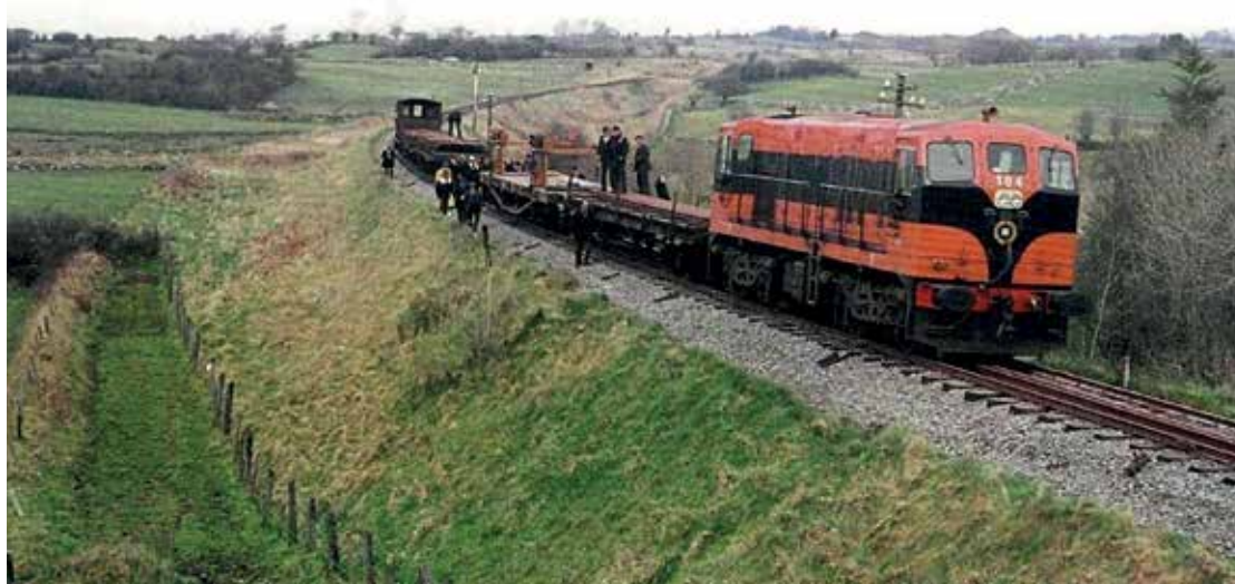
Figure 4.8: In March 1975 sections of rail in reasonably good condition were lifted between Kiltimagh and Swinford and exchanged with worn out rails from elsewhere. Closure would follow nine months later (Barry Carse).
