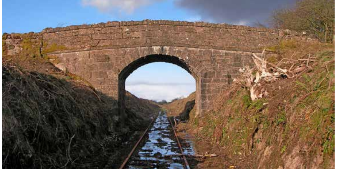
Figure 7.8: View south through cutting towards MP 36.50 and Carramore bridge showing severe drainage problem before remediation.
