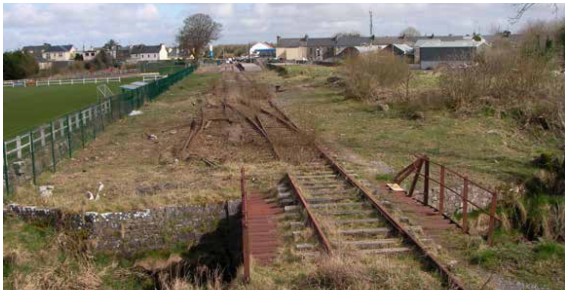
Figure 6.17 View east across Mullaghanoë River bridge from old signal post towards milepost 24.00 & Charlestown station. Turnout to the loop on the down side is just beyond the bridge.
