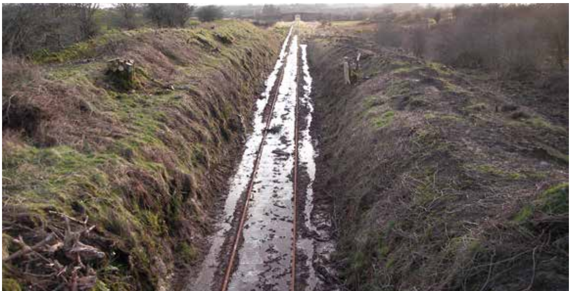
Figure 6.29 View south towards Carramore bridge (266) showing a severe drainage problem before remediation.
