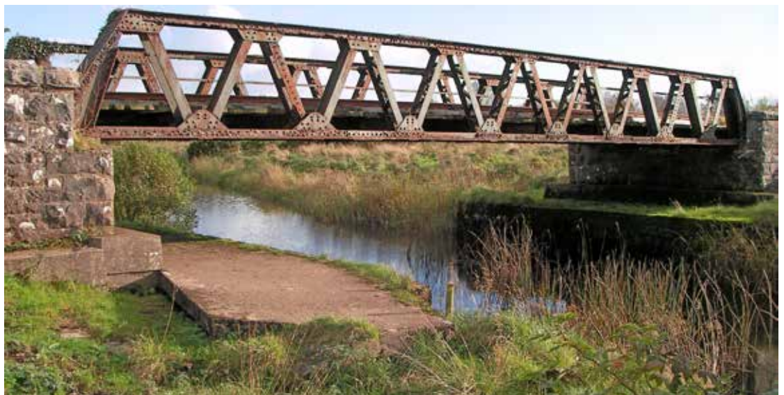
Figure 7.5: Single span Warren truss steel Girder Bridge crossing the Yellow River
