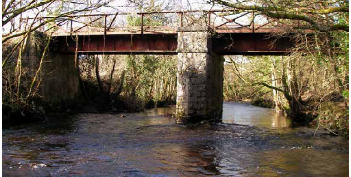
Figure 6.36: Southeast side of trough girder steel Owenbeg River bridge (273) milepost 42.00.
