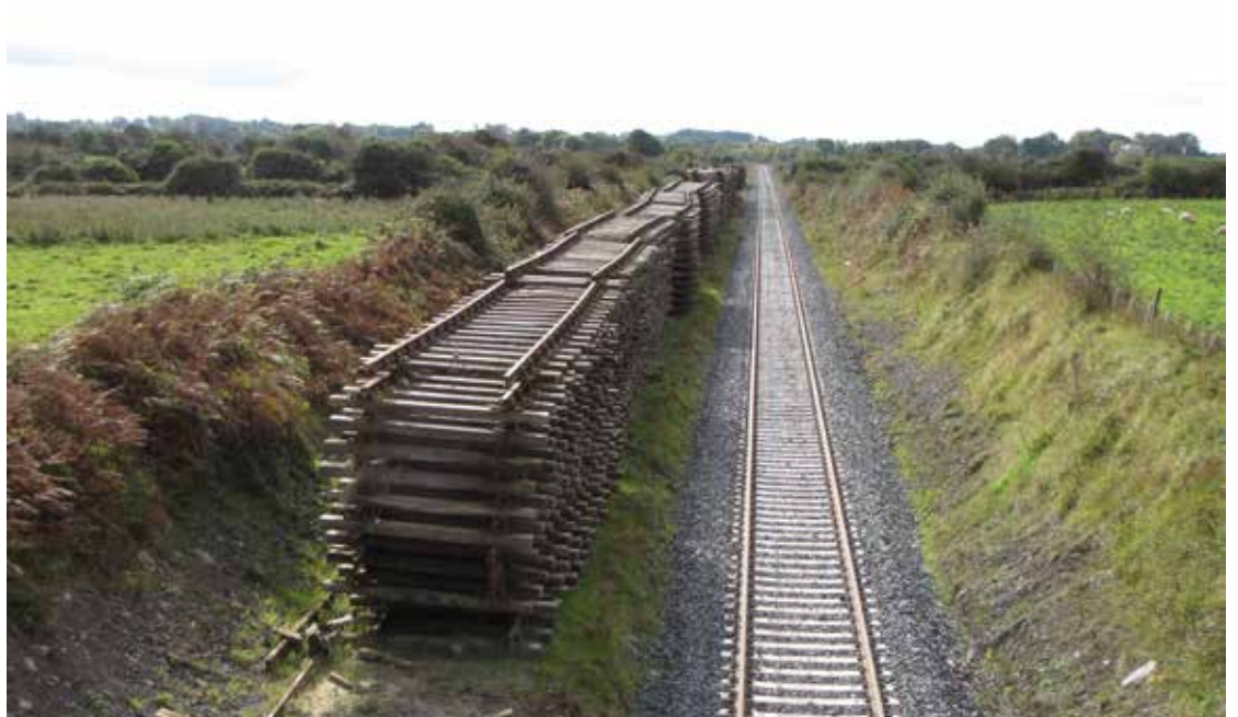
Figure 5.2: The newly constructed Athenry-Ennis railway with redundant track stacked alongside for disposal (David Dawson).
