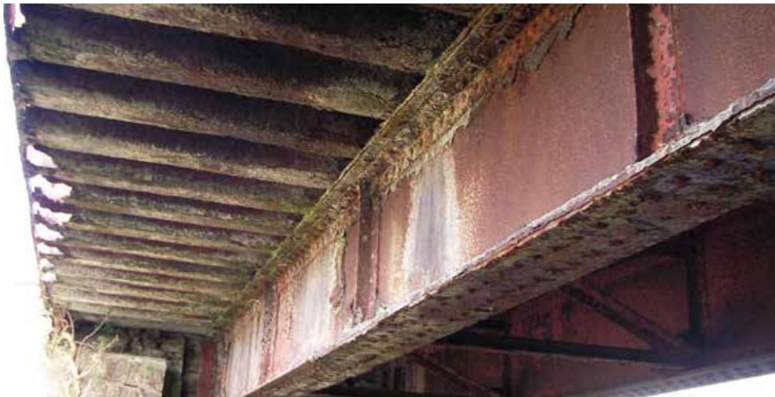
Figure 7.6: Underside of deck of trough girder steel Mullaghanoe River bridge
